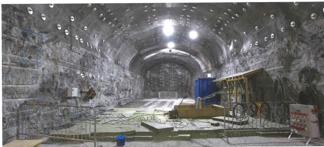
Above: ONKALO in Finland is slated to be the world's first operating deep geological disposal site
